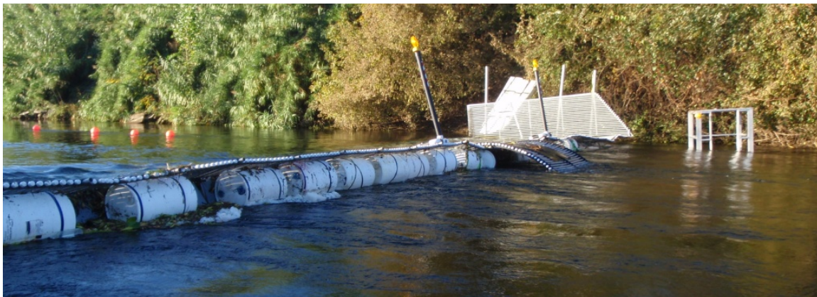
Figure 5. Photograph of the flotation barrels lining the underneath of the resistance weir.
