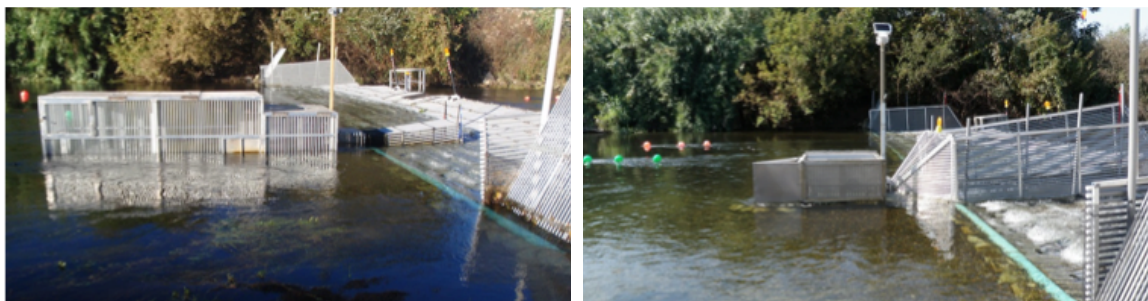
Figure 2. Tuolumne River Weir upstream trap and camera box before modifications (left photo) and camera box (upstream trap removed) after modifications (right photo).
