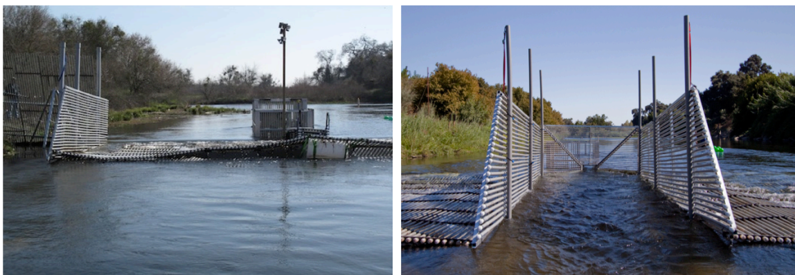
Figure 4. Tuolumne River Weir passage chute before modifications (left photo) and after modifications (right photo).
